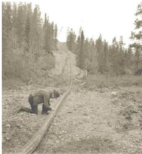
The 10 cm diameter Canol Pipeline (photo source Wikipedia)
